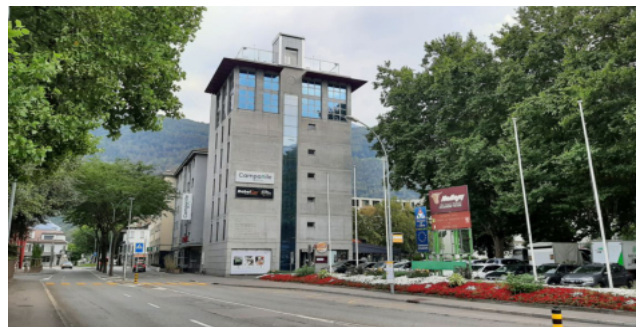
Hotel Campanile in Martigny
